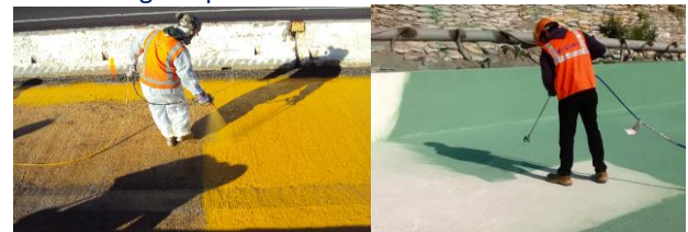
SPRAY APPLIED WATERPROOFING
